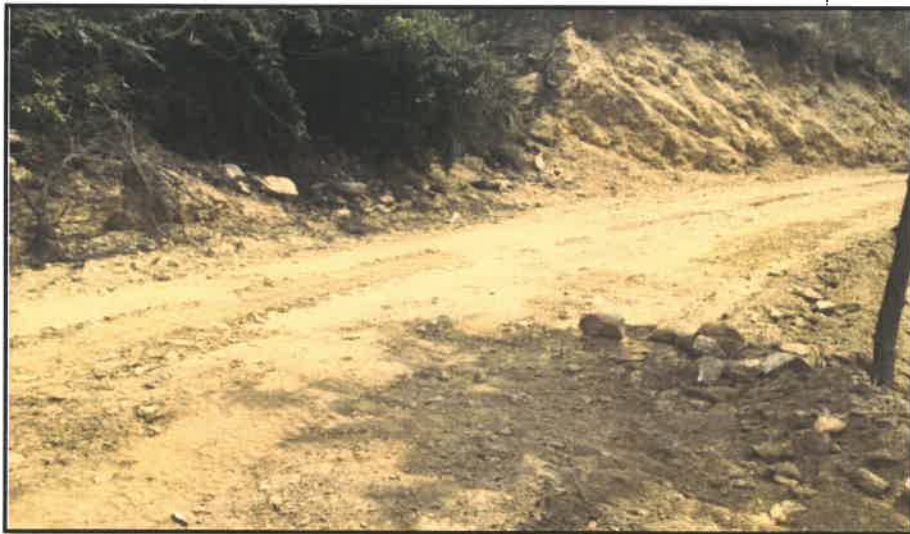
MATERIAL GRANULAR KM 0+500
