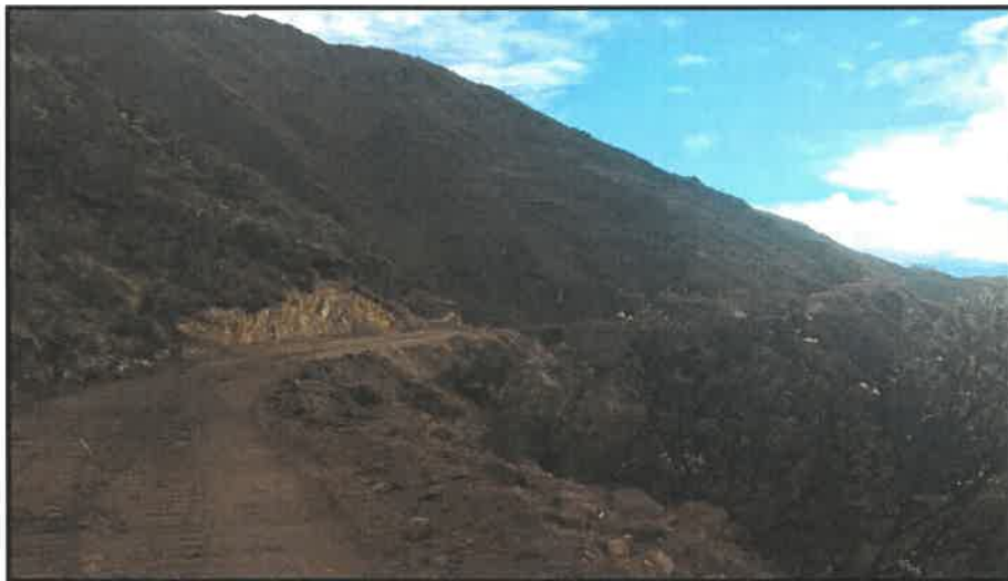
MATERIAL GRANULAR KM 10+500
