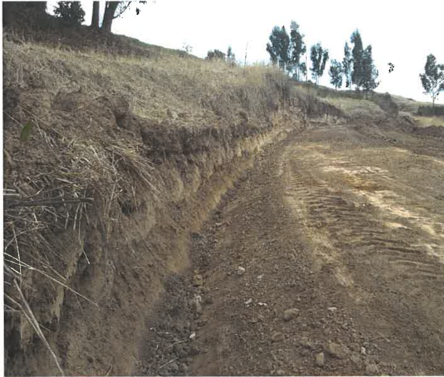
CUNETA RECONFORMADA KM 3+700
